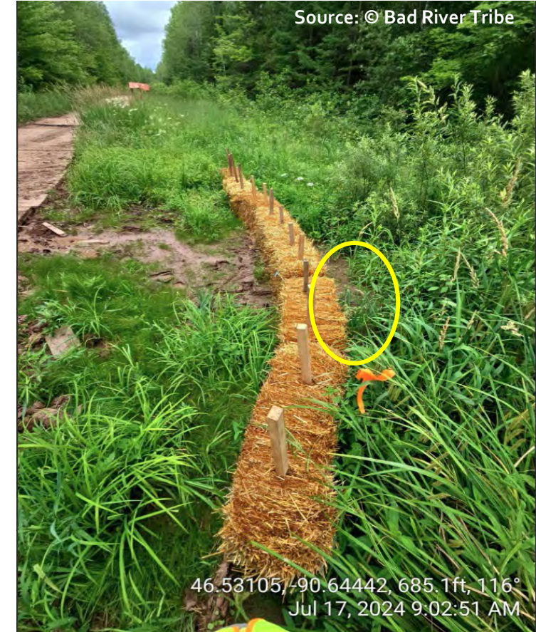
Enbridge Check Valve Project. Sediment both sides of straw bales. BMP either not implemented prior to sediment runoff or not installed correctly (2025, MNRD).
