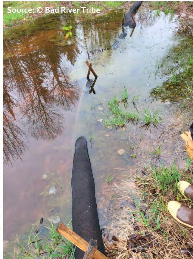
Photo of wattles/biologs placed along the access to the Check Valve site underwater during an April 2025 site inspection.
