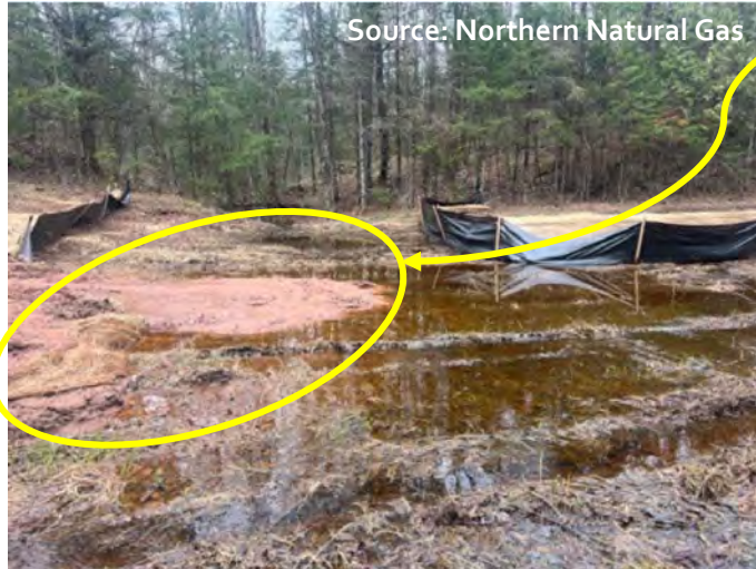
Northern Natural Gas BMP failure from sheet erosion. Soils and sediments reached a wetland downslope (left photo) and impacted the stream running through the wetland (right photo). Photos from Spring 2025.
