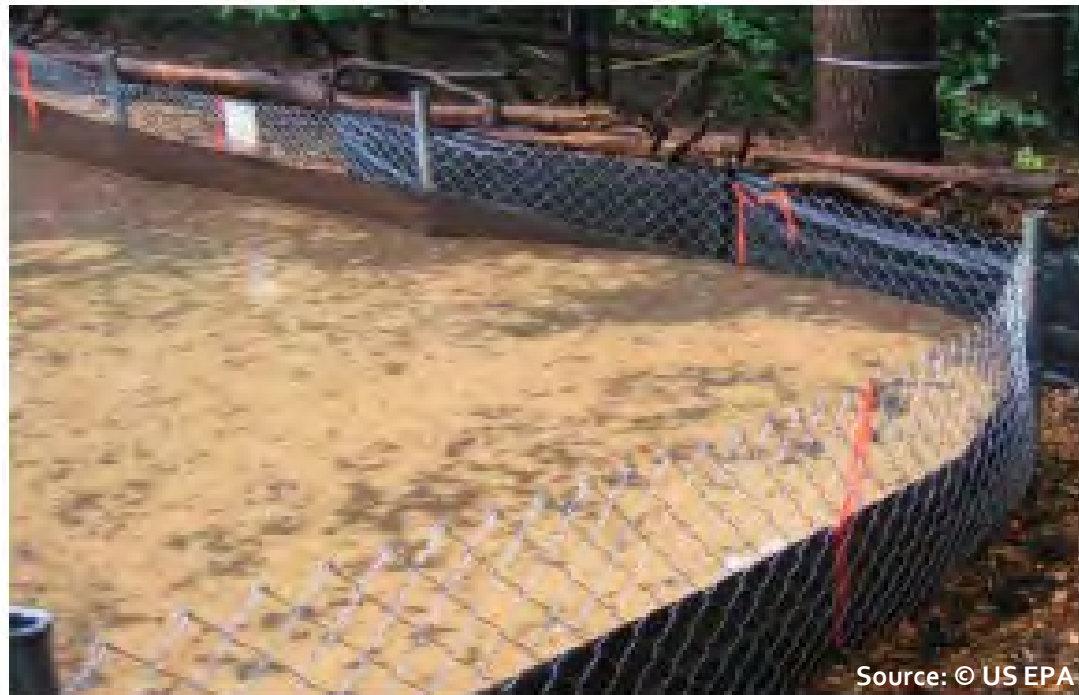
Image from US EPA NPDES: Stormwater Best Management Practice – Silt Fences shows chain link supported silt fence holding back runoff about to overtop the silt fence.
