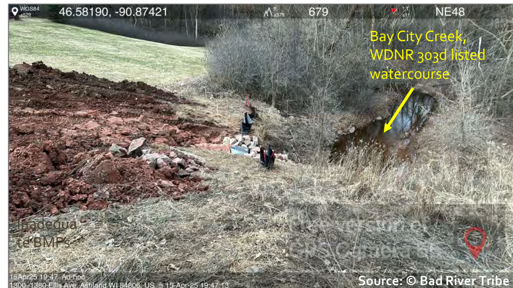
Inadequate installation of BMPs; WDOT project "WIS 13, Butterworth Road to US 2" (2025, MNRD).
