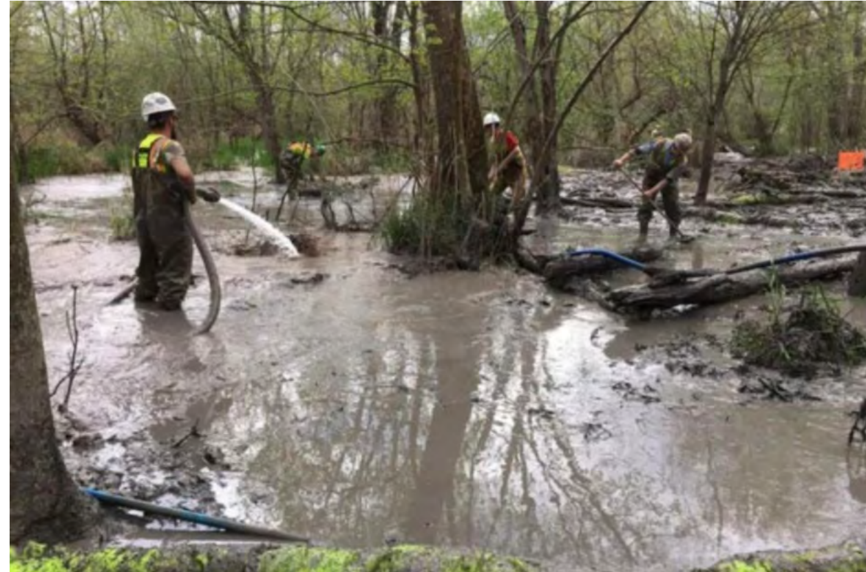
Will Affect Letter, Figure 3. Source: EPA, 2017. HDD inadvertent release – Tuscarawas River, Ohio.
