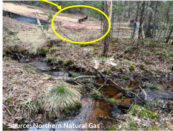
Northern Natural Gas BMP failure from sheet erosion. Soils and sediments reached a wetland downslope (left photo) and impacted the stream running through the wetland (right photo). Photos from Spring 2025.
