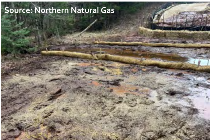
Northern Natural Gas failure from sheet erosion after additional BMPs installed. Wattles between the disturbed wetland and the stream channel (left) and silt fence with new straw bale support (right). Photos from Spring 2025.
