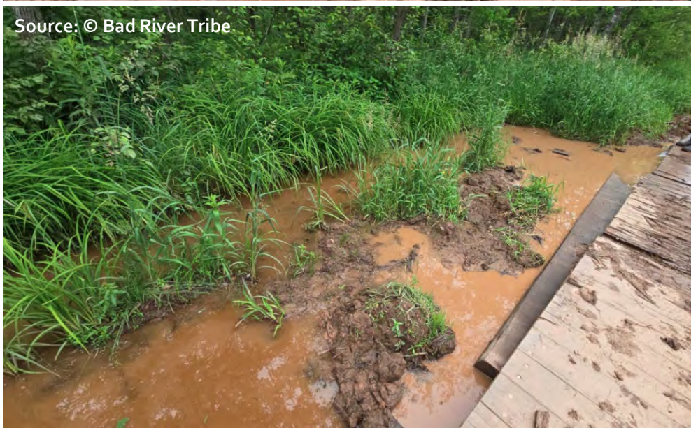
Timber matting along access roads does not eliminate soil disturbance.
