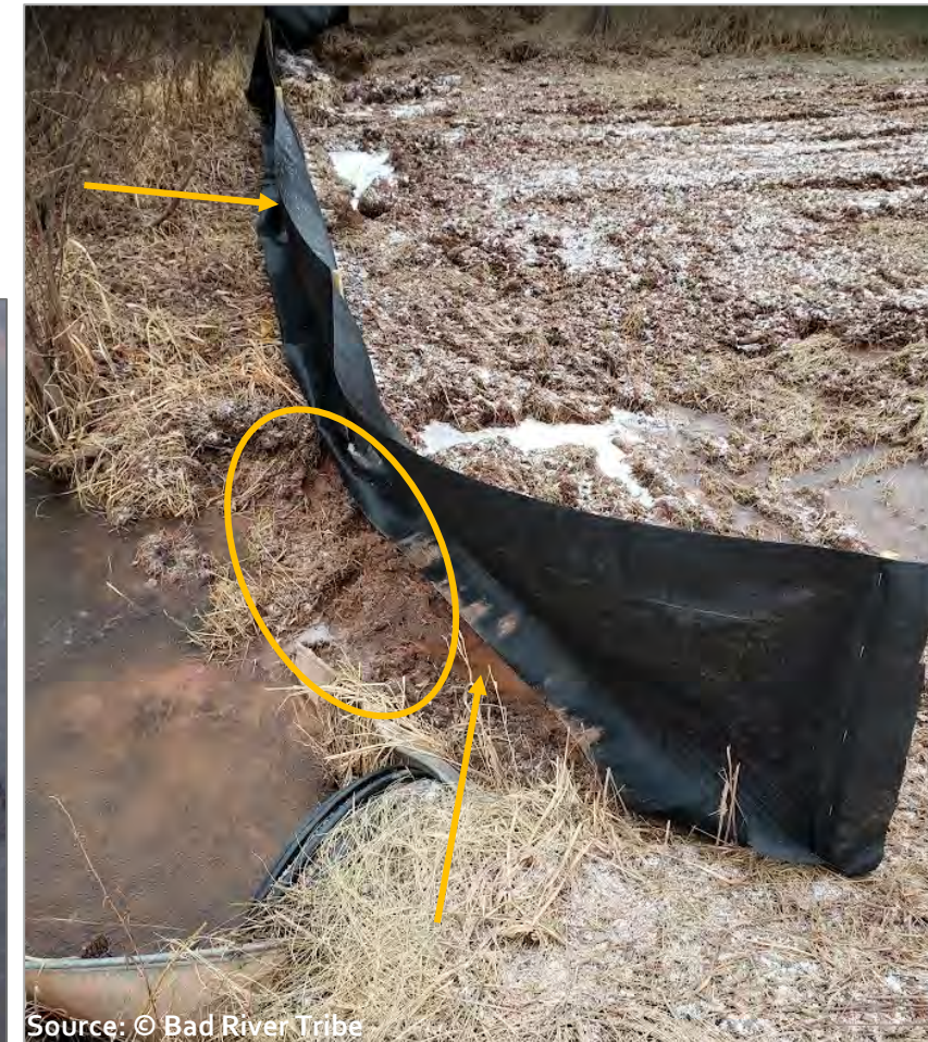
Incorrectly installed silt fence at an active construction site (2020, MNRD).
