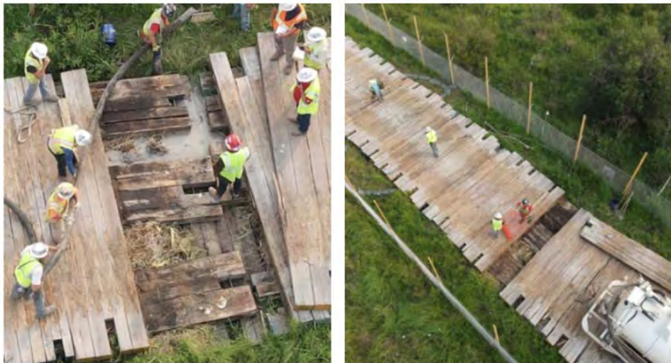
Figure 2. Drone photos of Enbridge clean-up crews trying to contain drill mud released under temporary matting associated with the HDD of the Mississippi River. Photos from Ron Turney included in Attachment 2 of Triplett-Dolph-Turney-Broberg Line 3 Fluid Losses and Aquifer Breaches.
