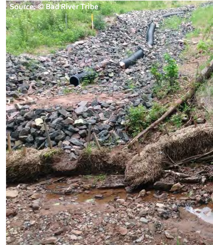
Photo of filled sediment basin and failing secondary straw bale containment in a Denomie Creek Tributary. Photo from 7/2021.
